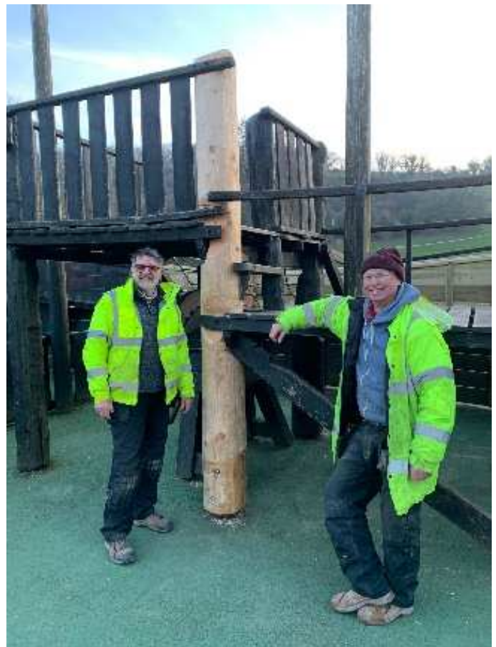
Steve Darbyshire gathers a crew to work on rebuilding the flagging Shamrock
