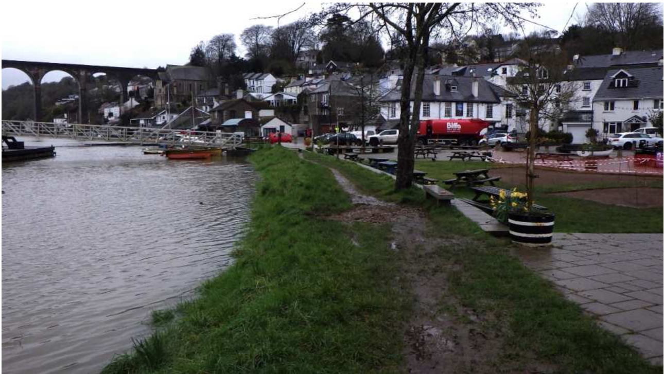
The biggest tide of the year on the 12th March - on big tides, water levels in the river are within 600mm of the top of the floodbank
